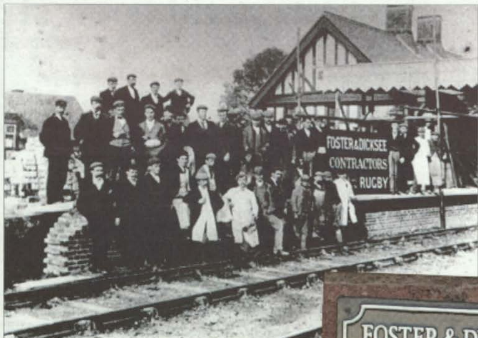
LEFT This picture shows workers from Rugby building firm Foster and Dicksee after building the railway station in Wolferton, on the royal estate in Sandringham. (s)
